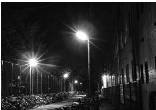
LED照明防犯灯
