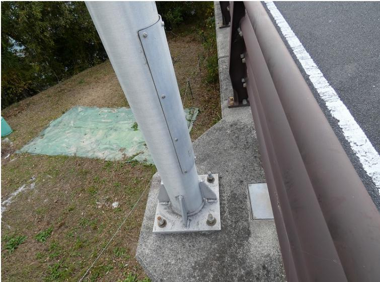
A close-up photograph of the base of a street lamp pole. The pole is made of galvanized steel and is mounted on a concrete foundation. The foundation is secured with several bolts. To the right of the pole, there is a metal plate on the concrete. In the background, there is a road with a white line marking and some greenery.                         | 大芝大橋電気設備<br>既設状況踏査<br><br>道路照明設備 |
